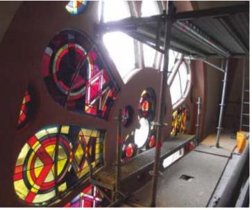
To protect these important and valuable works of art from weather and vandalism, a protective glazing is essential. The protective glazing consists of insulating glass with thermal protection and safety glass (VSG) to prevent the condensation.
